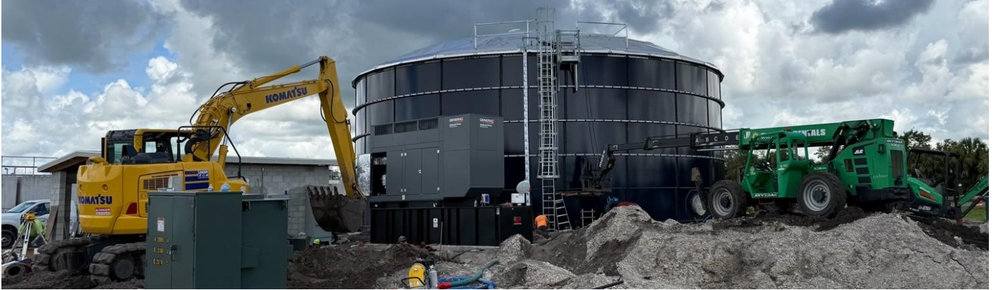
0.5 MG potable-water storage and 2,500 gpm booster pump station under construction
