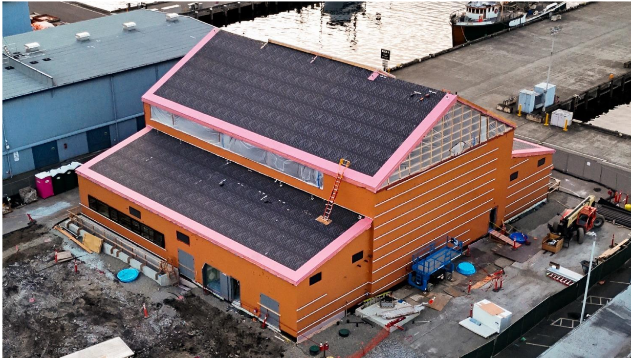
Maritime Innovation Center under construction at Fishermen's Terminal in Seattle
